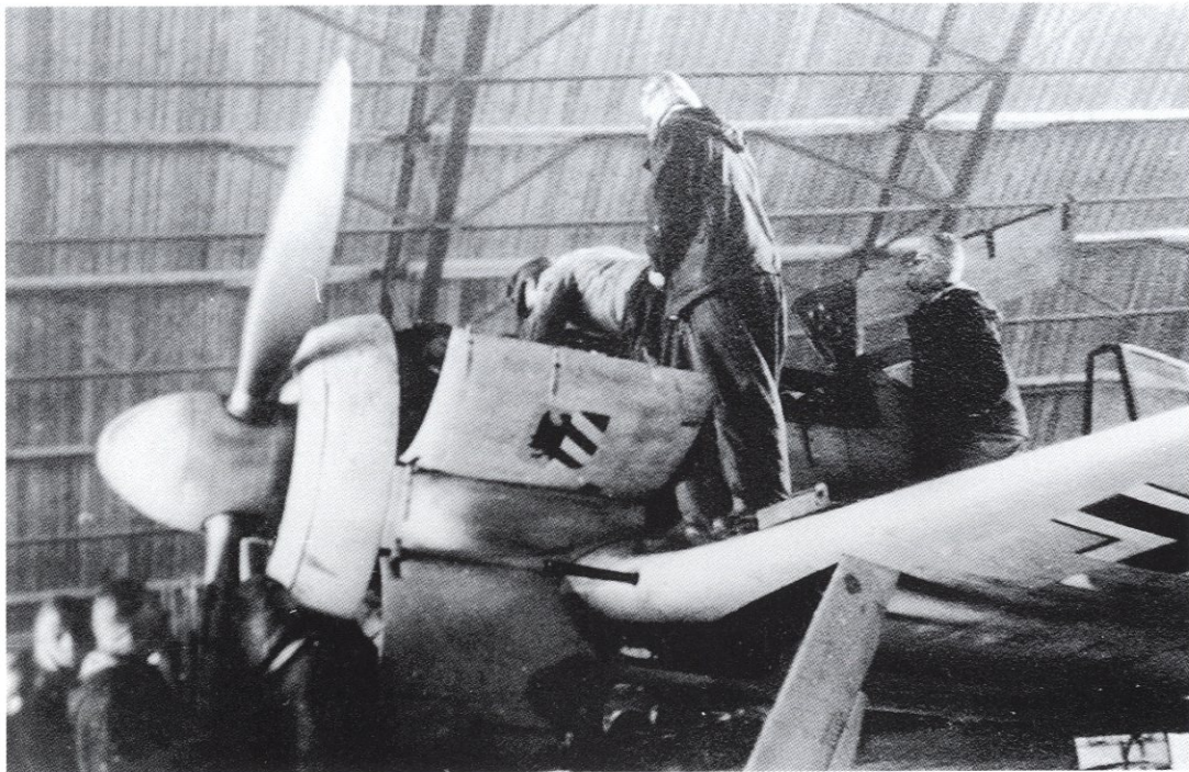
LEFT: This Fw 190 A undergoing maintenance at Siwerskaja has had its outer wing guns deleted. Pilots reported that the ammunition feeds to these weapons sometimes jammed due to g-forces during high-speed manoeuvres, but the main reason for deleting them was to save weight and therefore improve the aircraft's speed and manoeuvrability.
