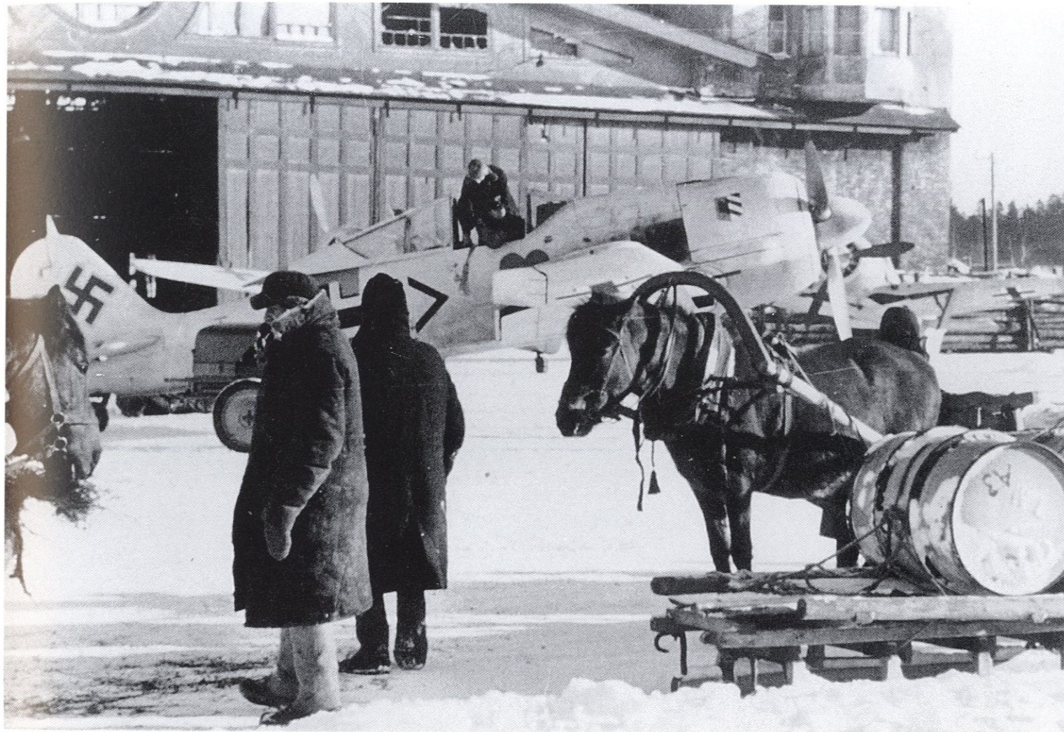
LEFT: This Fw 190 A undergoing maintenance at Siwerskaja has had its outer wing guns deleted. Pilots reported that the ammunition feeds to these weapons sometimes jammed due to g-forces during high-speed manoeuvres, but the main reason for deleting them was to save weight and therefore improve the aircraft's speed and manoeuvrability.
